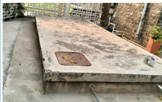
Rain water storage tank
