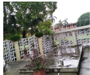
Rainwater storage tank
