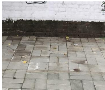
Paving Stone Installed in Campus
