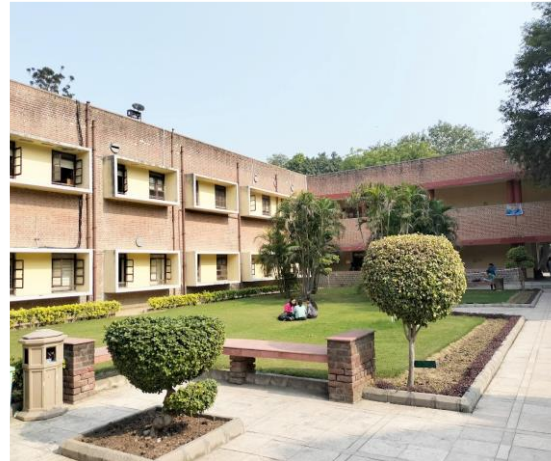
Well ventilated building
