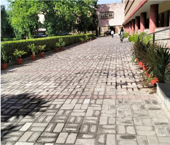
Paving stone installed in campus
